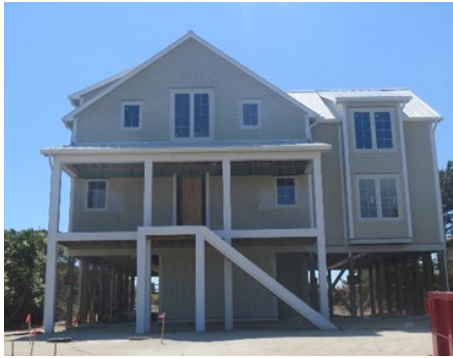
Figure 2.7. Post and beam/piling
