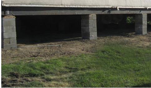
Figure 2.1. Ineligible dry-stack foundation
