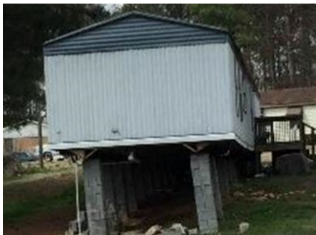
Figure 2.2. Ineligible dry-stack foundation
