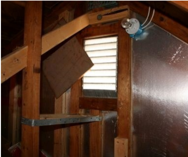
Figure 3.2. Example of a gable end vent
