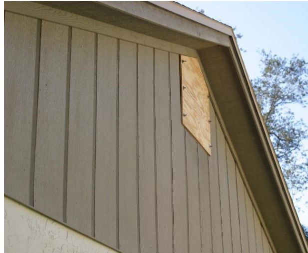
Figure 3.3. Outside shuttering of a gable end vent with Plywood
