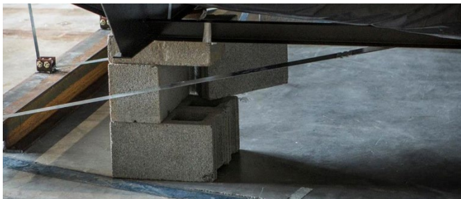
Figure 2.3. Ineligible dry-stack foundation
