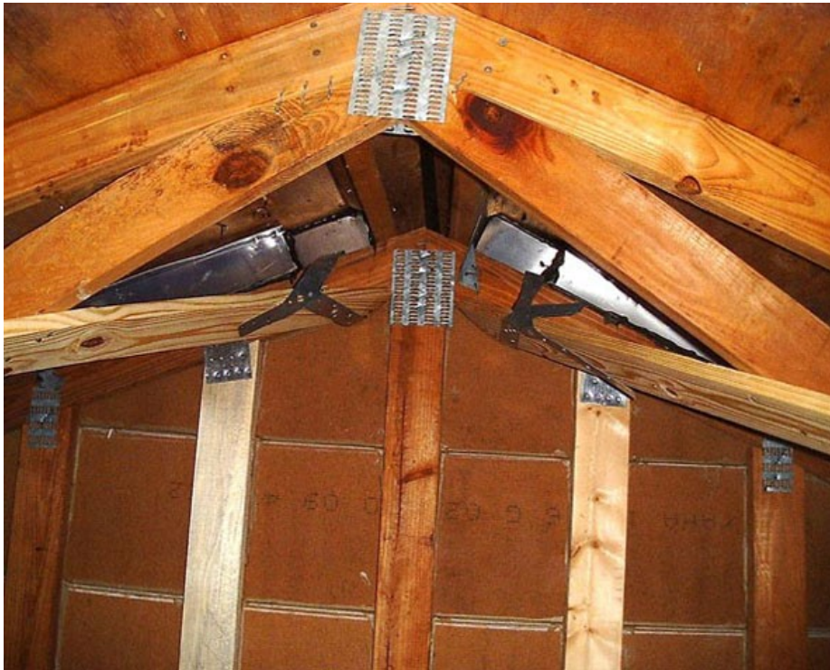
Figure 5.2. Blocking of gable rake soffit vents using metal flashing
