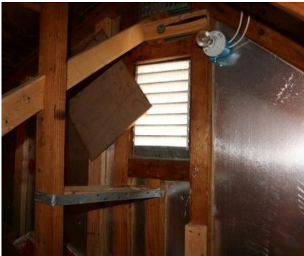
Figure 3.2. Example of a gable end vent with
