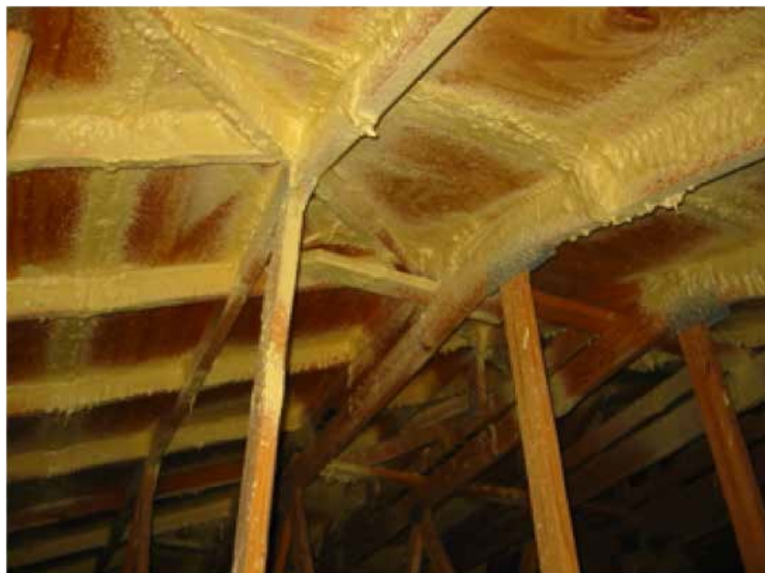
Figure 3.1. Closed-cell polyurethane foam adhesive applied to underside of roof sheathing
