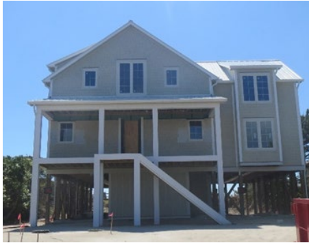
Figure 2.7. Post and beam/piling
