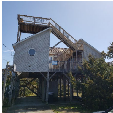
Figure 1: Wood Framed Deck built over the roof area of a home
