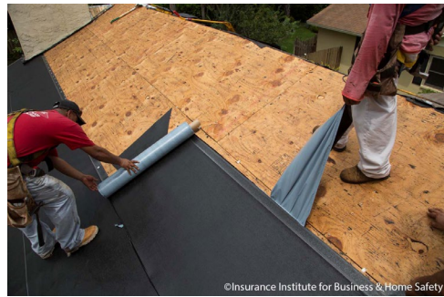
Sample Photo 4: Underlayment "peel-and-stick"
