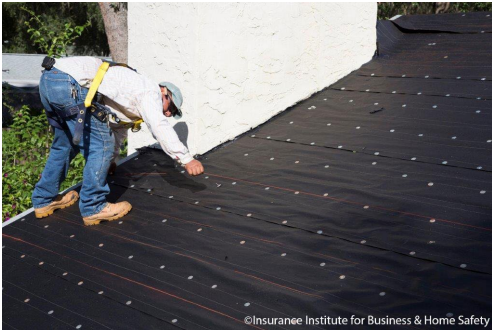
Sample Photo 3: Underlayment Nailing
