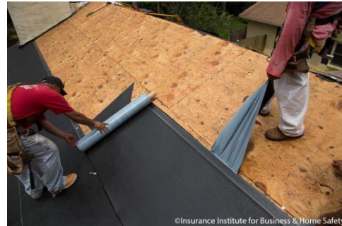
Sample Photo 4: Underlayment "peel-and-stick"
