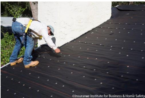
Sample Photo 3: Underlayment Nailing
