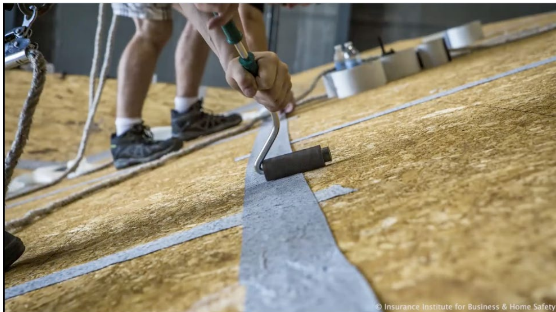
Figure 3. Installing a sealed roof deck system; taping the seams of roof sheathing.
