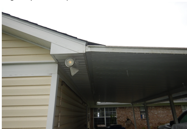
Figure 3. Example of accessory roof that meets main roof at eave.
