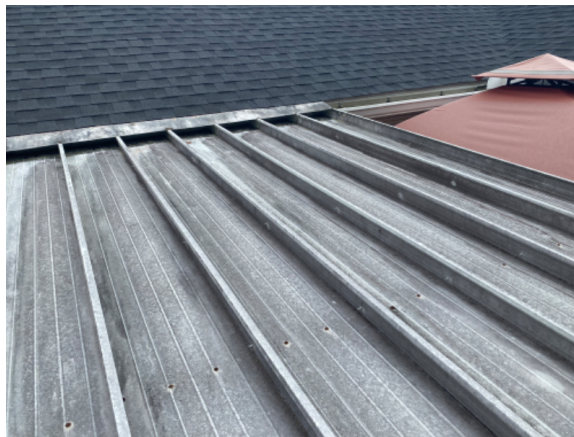
Figure 4. Example of accessory roof that meets main roof at eave.
