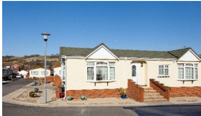
Figure 2: Example of stairs on home built to the HUD Code
