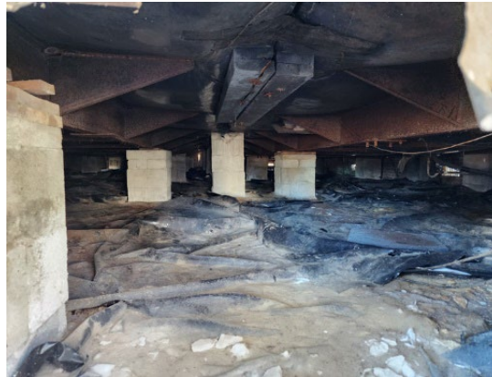
Figure 3: Example of metal chassis of home built to the HUD Code
