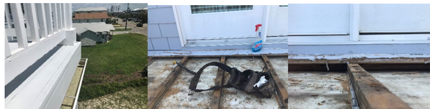
Figure 2: Framed Deck located on a flat roof over living space
