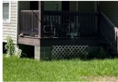
Figure 9. Post and beam/piling.
