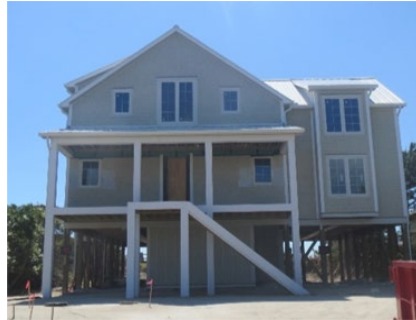
Figure 7. Post and beam/piling
