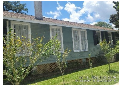
Figure 8. Post and beam/piling
