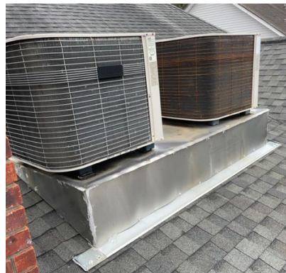
Figure 2: Metal support frame over the roof area of a home
